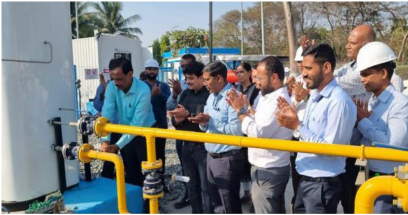
Figure 3: Kawas HoP P Ram Prasad starting the green hydrogen injection into PNG network of NTPC Kawas Township
